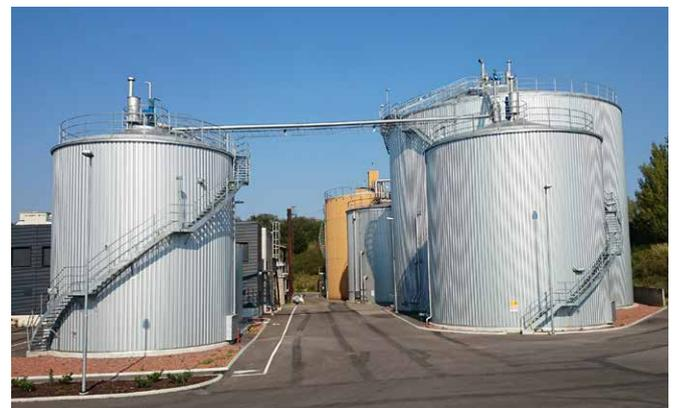
**Figure 3:** The blending tank to the left and the digester and post-digester tanks to the right.
